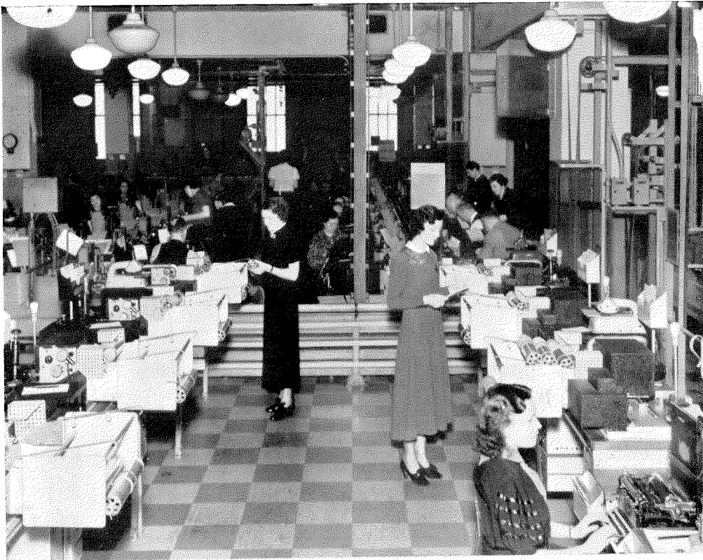
Fig. 13—Operating room in New York showing some of the facsimile equipment employed on long-distance trunk circuits.
